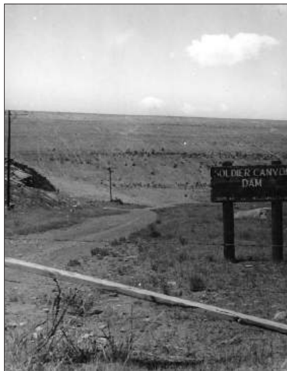
Figura 64 - La Soldier Canyon Dam, U.S. Bureau of Reclamation, Fort Collins, Colorado (foto R.J., 1953).
